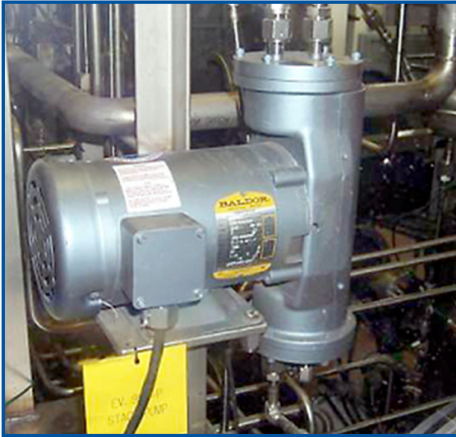
Metal bellows pump. Photo: US ITER
